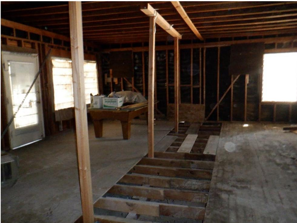
Plate 37. Support beams recently added, looking north. Interior photo taken on August 14, 2020.
