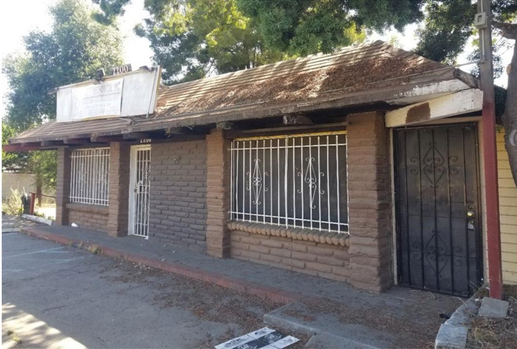
Plate 34. West façade with adobe brick veneer and faux rafters, looking northeast.
