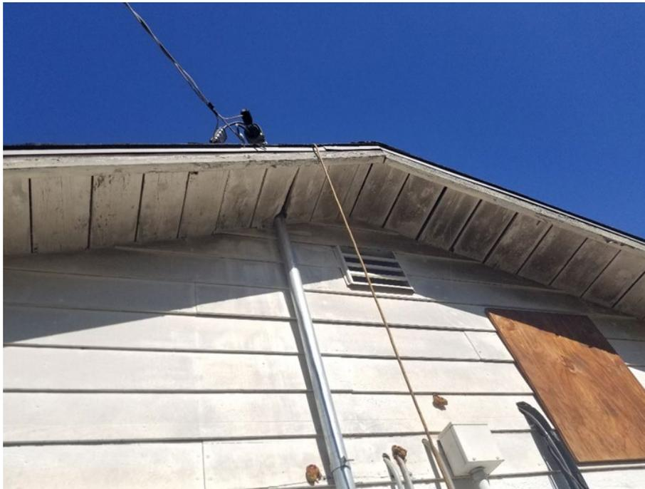
Plate 50. East façade of 1940s portion with ship lap wood siding and front gabled roof, looking northwest. Photo taken on July 9, 2020.
