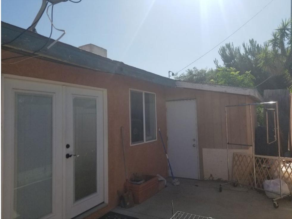
Plate 51. South façade with stucco clad enclosed breezeway addition and French doors, looking southeast. Notice the vertical wood boards that clad the original 1947 portion.
