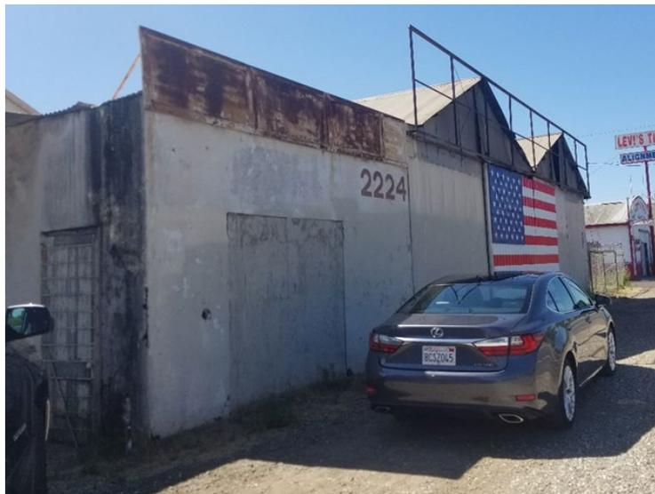
Plate 20. Welding shop, looking southeast. Notice the early wood shop with stucco siding attached to the corrugated metal addition from the 1940s. Photo taken on July 9, 2020.
