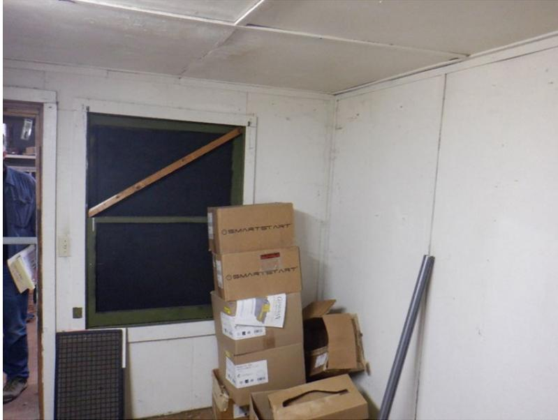
Plate 44. Interior of addition on the south façade, looking north. Notice the original exterior wood window frame that was enclosed when this addition was added, looking north.
