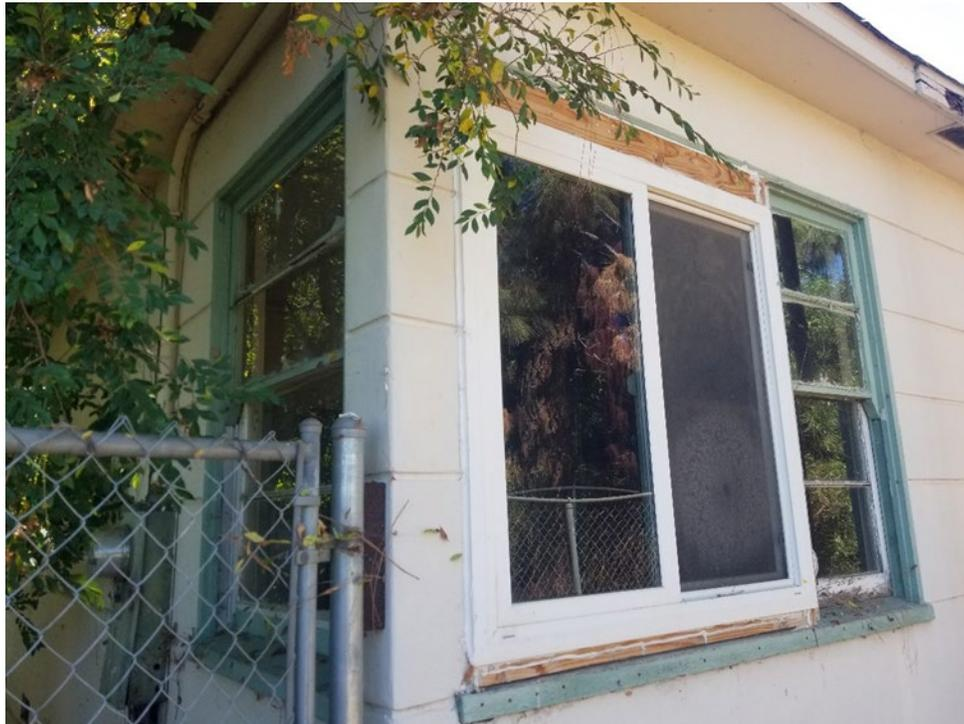
Plate 30. Northwest corner of the dwelling with original windows on the north façade and a combination of contemporary vinyl sliding window with an original double hung window on the west façade, looking southeast. Photo taken on July 9, 2020.
